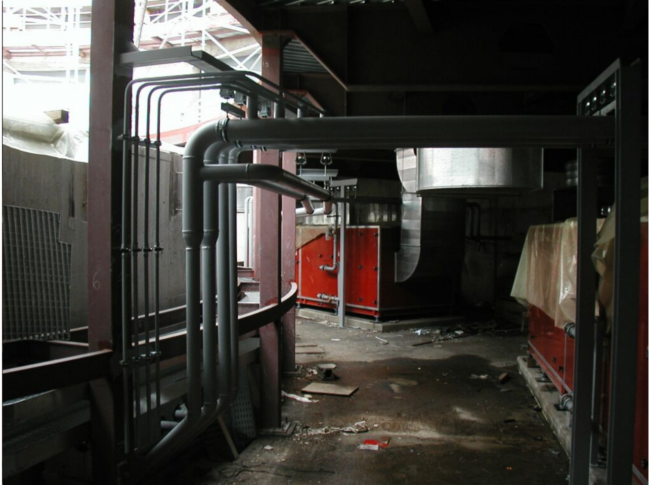
Fig. 3. Inside the GTC dome. Many complicated systems are required for the operation of the GTC. Some of the cooling subsystems are seen here.
