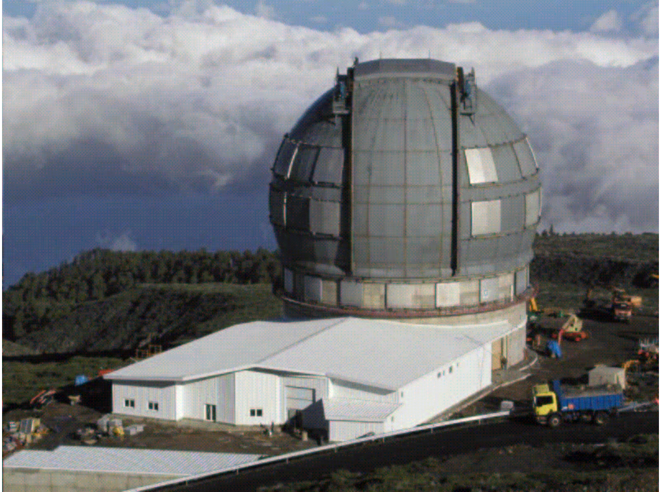
Fig. 2. Current view of the building site. Note that both the dome and building are nearly completed.
