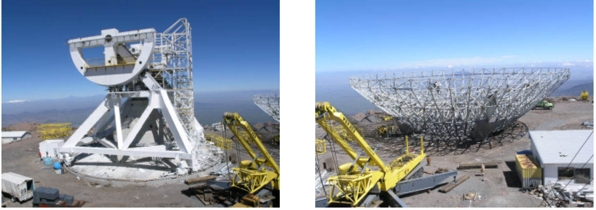
Fig. 1. Left: The LMT azimuth-track, bogies, alidade, ballast cantilevers and receiver cabin (open-frame structure) are nearing completion before the installation of the antenna. Right: Backing-structure of LMT antenna. In the foreground one of the two 1000-ton cranes required for the lift of the antenna onto the elevation mount (to take place in September 2005) is being prepared.
