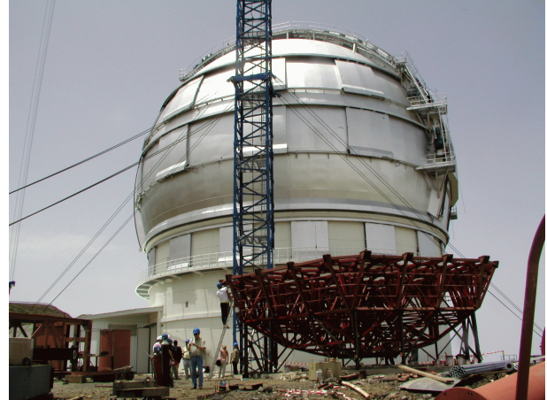
Fig. 3. A view of the GTC dome with the supporting cell of the primary mirror in the foreground, soon to be integrated in the telescope structure.
