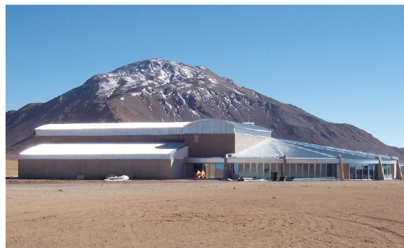
Fig. 3. The ALMA Technical Building on Chajnantor.
