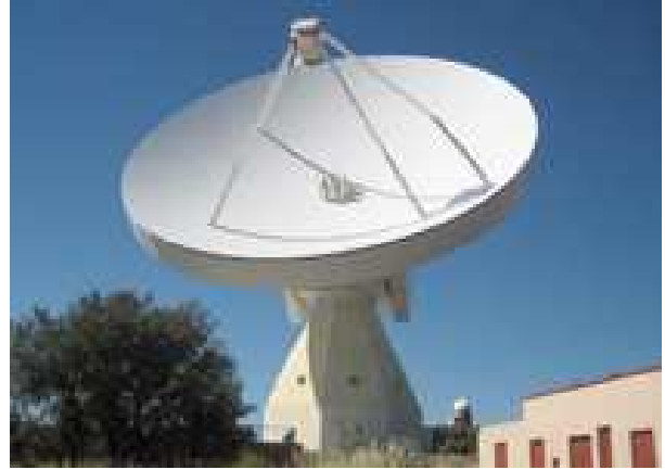
Fig. 3. Communication Antena, 30 m size, located in Tulancingo, Hidalgo, México.
