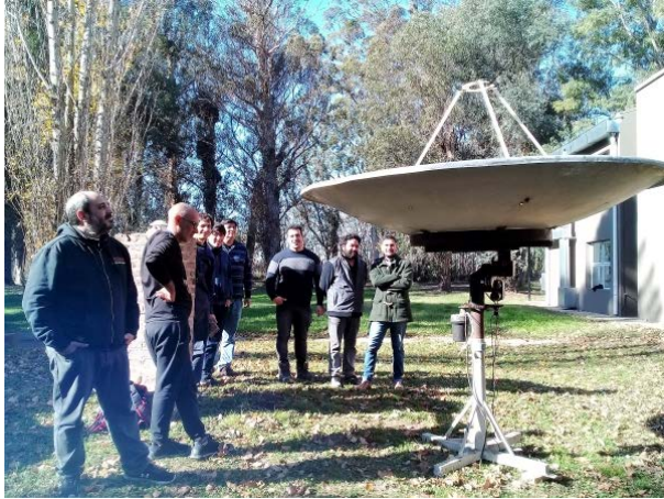
Fig. 28. Martín Salibe, Leandro García, Santiago Spagnolo, Luis Ferruffino, Juan M. González, Matías Contreras and Darío Capucchio after the Ground Station Prototype installation.
