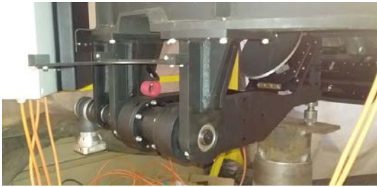
Fig. 7. M1A mirror assembly installed at the bottom of the CASS structure.
