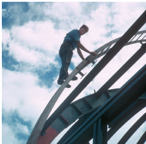
Fig. 1. Stock climbing girders for a CIDA dome in 1972. The girders for three domes were intermingled without markings and had to be assigned to their domes by trial and error. He called it his biggest ever 'rompecabezas'. Photo by A. G. D. Philip.
