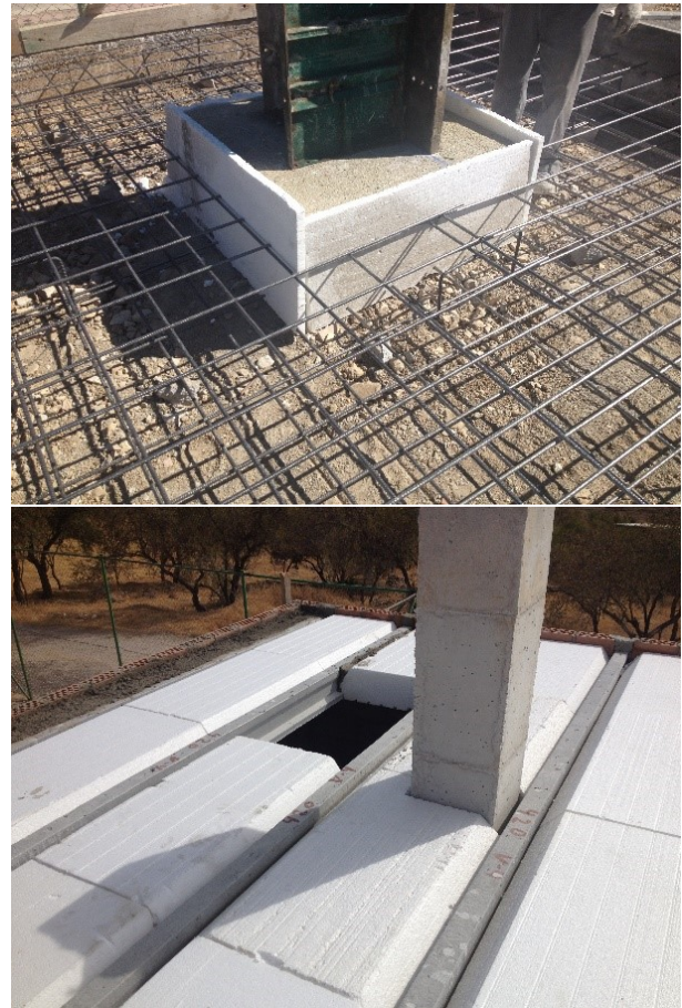
Fig. 2. Detail of the foundation of the pillar and structure. It can be seen how the pillar and its foundation slab are totally isolated from the rest of the structure of the building.
