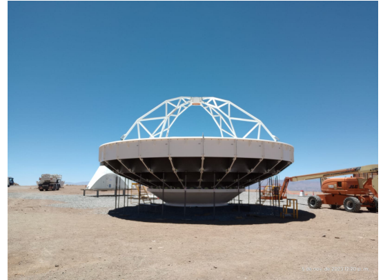
Fig. 1. The dish of the LLAMA Radio Telescope being mounted.
