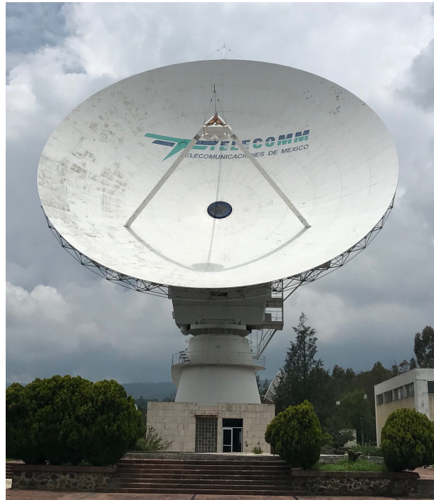
Fig. 1. Front view of the 32-m Tulancingo-1 antenna. The electro-mechanical work for the conversion to a radio telescope is largely complete; commissioning will commence in 2024 using an L-band receiver.
